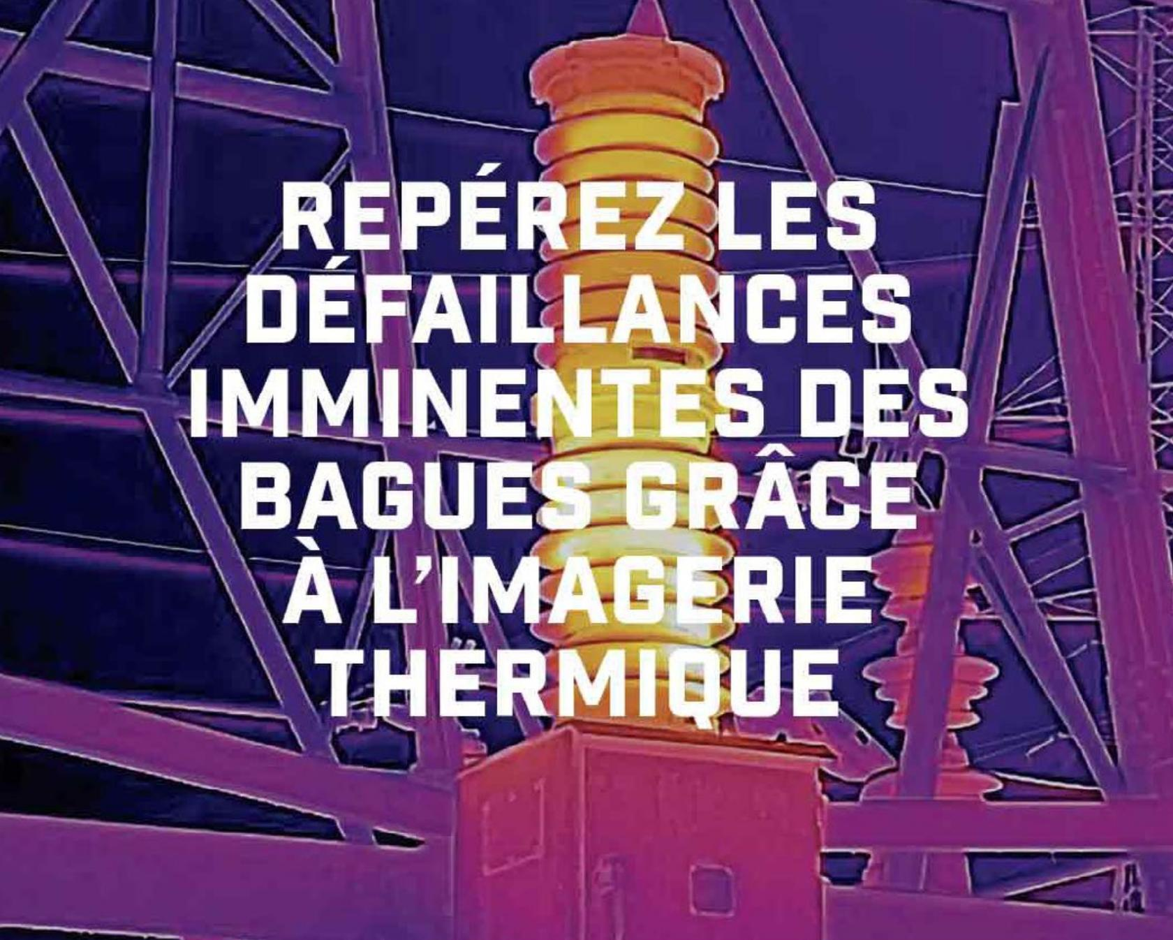
A thermal image of a power line tower. The central bushing is highlighted in bright yellow, indicating a hot spot. The rest of the tower and surrounding structure are in shades of purple and blue, indicating lower temperatures.
